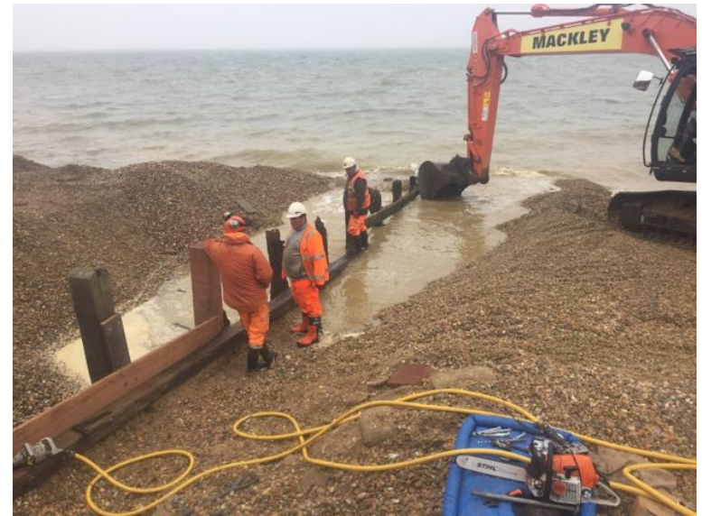
Phase 1: Urgent beach and timber works
